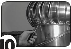
After installing, check to see that Whirlybird® turbine vent turns freely. In transportation it may have shifted slightly. If necessary, minor adjustment may be made by gently prying lowest point of turbine upward to remove any wobble.
