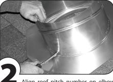
Align roof pitch number on elbow Place 3 screws through holes that line up tapping roof. with predrilled holes in base.
