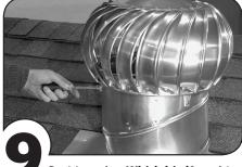
Position the Whirlybird® turbine head on the base. Line up the predrilled holes in the brackets and elbow and fasten with sheet metal screws.
