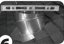
Rotate top of elbow to level position
