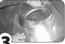
Locate base opening between rafters with the indicator line on the base flashing. and mark hole to be cut. Locate rafters by
