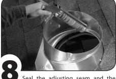
Seal the adjusting seam and the base/elbow connection seam on inside with roofing cement. Seal locking clamp holes and all exposed nails with roofing cement.
