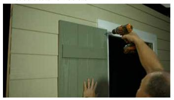
C. Remove the shutter and pre-drill pilot holes through the facade.
