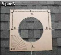
3. Use the supplied template to mark the hole location and shingles to be trimmed. Position the template vertical center mark (A) in line with the nail driven from the inside of your attic or air space. Position the template horizontal center mark (B) in line with the nearest bottom of a course of shingles. Mark hole position and shingle trim area. Also, mark the center position at the sides and bottom of template. See figures 3 and 4.
