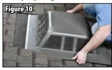
7. With the side marked UP aimed toward the ridge, carefully slide the unit into place allowing the motor wiring to hang down into the vent opening. Align the center marks on the flashing to the center marks made from the template, this will ensure that the throat of the unit is centered over the vent opening. See figure 10.
