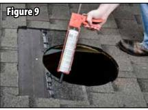
**6.** Apply roofing cement around the edge of the vent opening. **See figure 9.**
