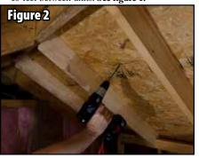
2. From inside the attic mark hole location by measuring down 24 to 36 inches from the roof peak centered between two rafters. Drive a nail or drill a screw through the roof at the confirmed location so it can easily be found on the roof outside. See figure 2.
