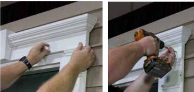
2c. When fastening the crosshead using exterior grade screws ensure that you slowly countersink the screws into the crosshead approximately 1/8", similar to screwing into drywall.
