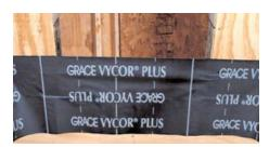
**Step 5** Install the sill piece of Vycor self-adhered flashing.
