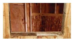
**Step 1**Prepare the rough opening. Remove dust, dirt and loose nails.
