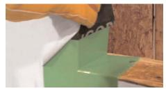
**Step 4A-2x4 construction**Install a piece of Vycor self-adhered flashing over the top edge of VYCORner at the rough opening. Extend over the face of VYCORner (underneath the WRB) a minimum of ½ inch. Repeat on both sides.
