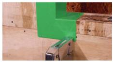
**Step 2** Position and attach VYCORner into place.
