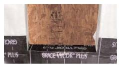
**Step 5**Install the sill Vycor flashing. Make vertical relief cuts and adhere to the sill.
