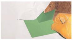
**Step 2**Insert VYCORner under the WRB to allow for proper drainage; repeat on both sides of the ill.
