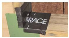
**Step 4B–2x6 or 2x8 construction**Install a patch of Vycor selfadhered flashing as shown in the photo – to extend a minimum 1 inch beyond VYCORner at the sill and jamb of rough opening. Repeat on both sides.
