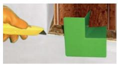
**Step 1**Make approximately 2.5 inch long horizontal cut in the WRB, starting from the corner.
