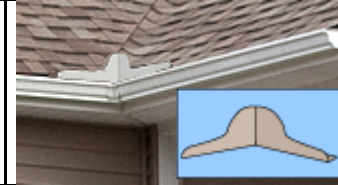
Splash Guard/Gutter Repair
